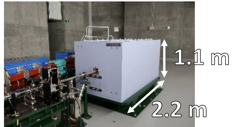
Beam dump (Steel)
