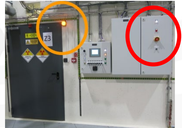
Door of the ring tunnel
