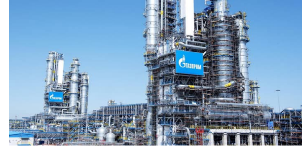
Explosion at Gazprom's Amur natural gas processing facility on 5th January 2022
