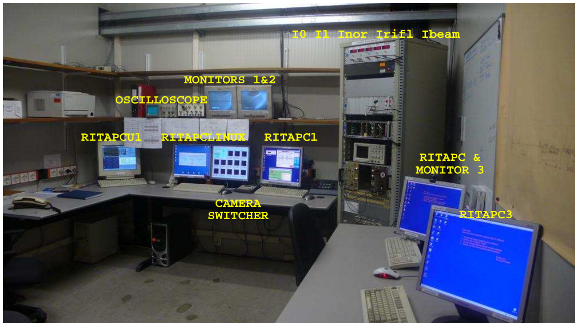
GILDA's control cabin
