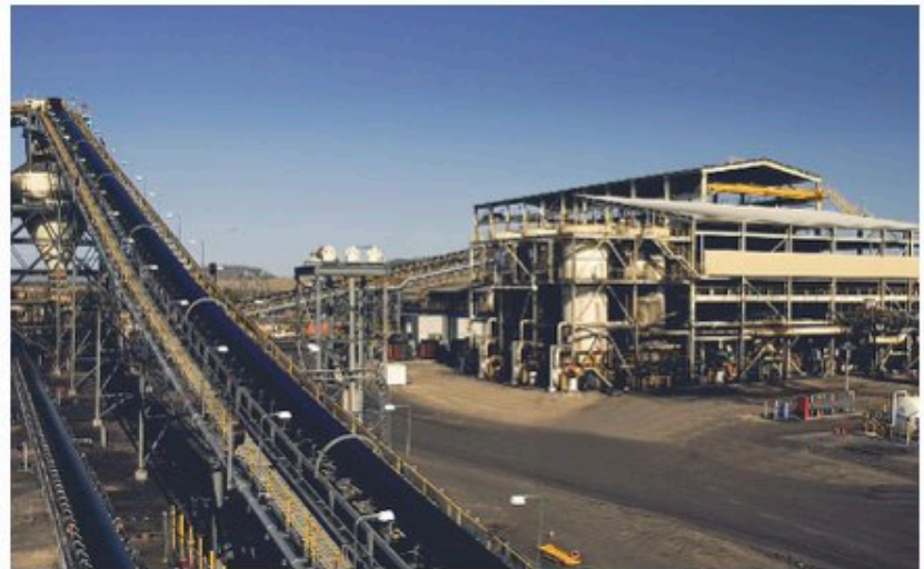
The Caval Ridge coal handling and preparation plant
