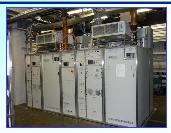
From 2007, the RF plant # 9 available power *is* 150 kW = max (80 kW + 80 kW) Combiner: WG switchless
