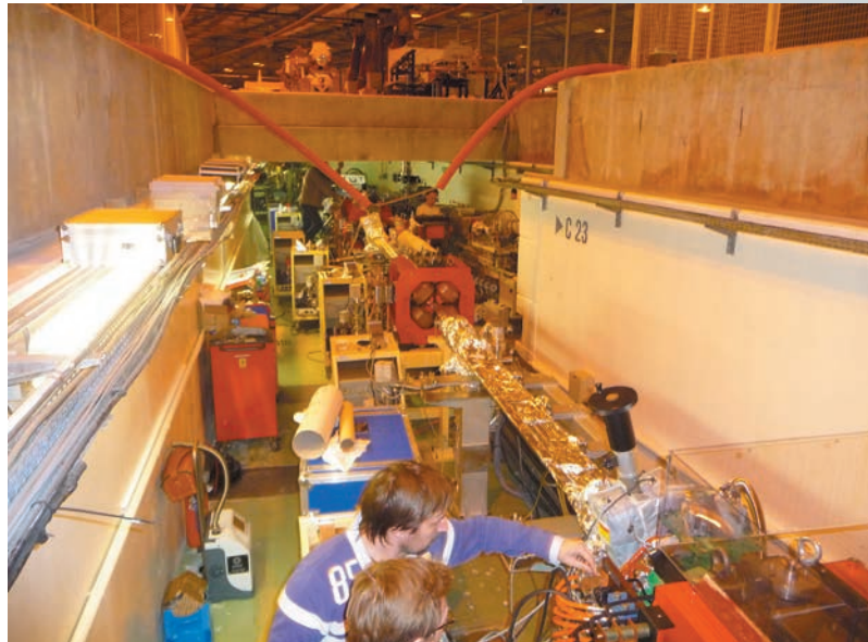
Fig. 162: The first 7 m straight section during installation at ID23 in January 2013.
